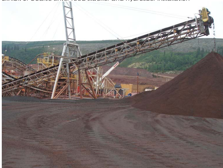
Exhibit 8: Coarse sinter feed stacker and hydrosizer installation
